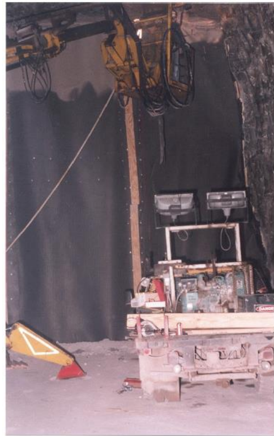
Figure 8. Fabric-grid material sprayed with cementitious material.
