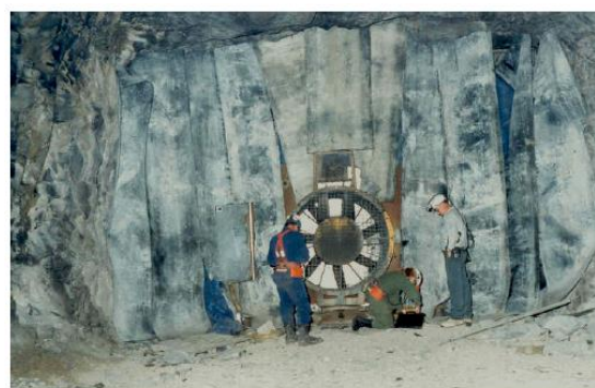
Figure 4. Used mine belt used pressure relief.
