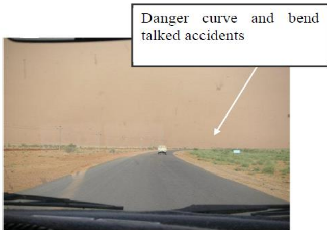
Figure 2. The width of the road and showing the narrowness of the width of the road and shows the separating line without pavements to the trajectories facing each other in direction also it shows that there is no light and no water sewage also the sides of the road are narrow. This picture has been taken from the Khartoum Medani road
