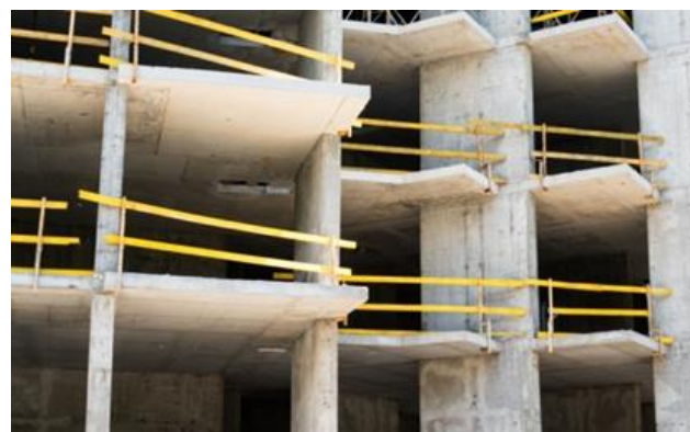
Fig2 Post-tension slab Source [reference 4]
